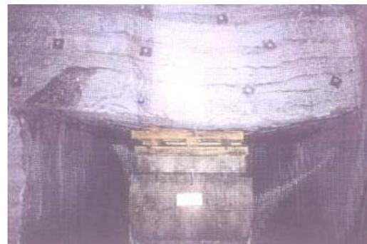
Figure 5: Example of separation of roof (source, MDP A 2015).
