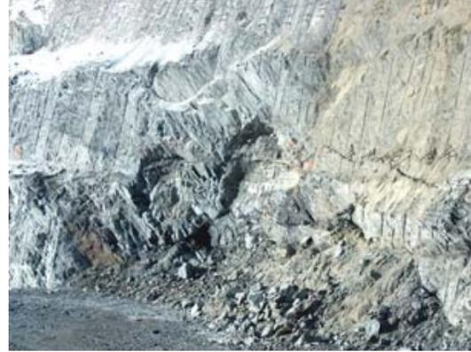
Figure 4: Pit wall undercut by stope.
