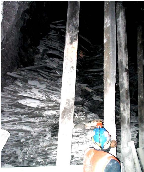
Figure 3: Typical roof fall showing laminated nature of the silty shale roof rocks and steep-sided collapse cavity.
