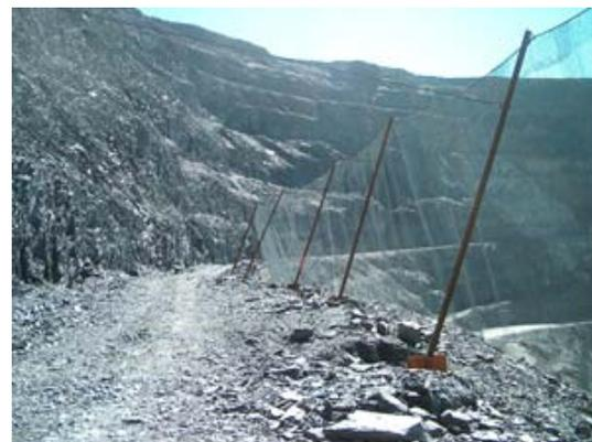
Figure 7: Catch fence installation along bench.
