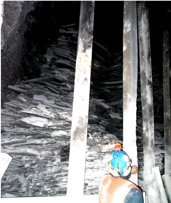
Figure 3: Typical roof fall showing laminated nature of the silty shale roof rocks and steep-sided collapse cavity.
