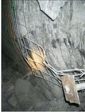
Figure 1: Foliated schistose rockmass in footwall buckling towards the drift (Case Study Mine).
