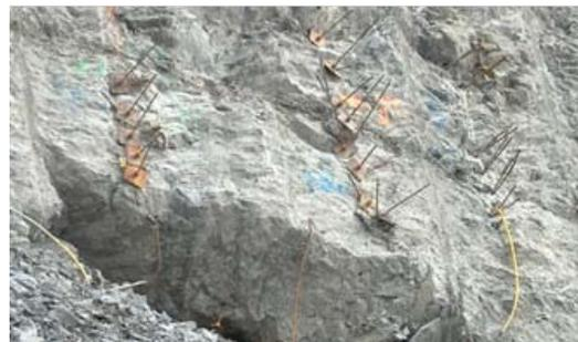
Figure 6: Cable bolt reinforcement above void in pit wall.
