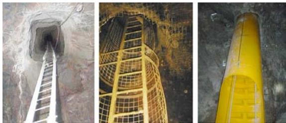
(a) Simple steel design (b) Steel cage (c) Laddertube
